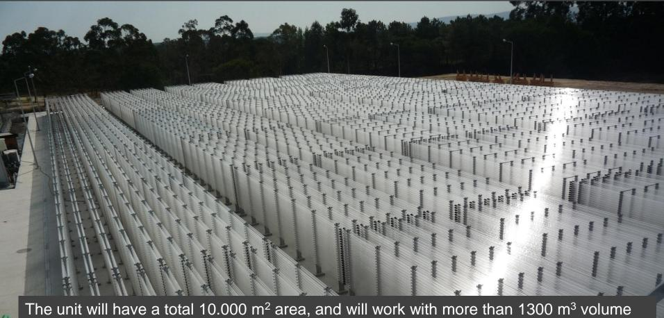
The unit will have a total 10.000 m<sup>2</sup> area, and will work with more than 1300 m<sup>3</sup> volume of production photobioreactors, being the world's largest unit of microalgae production with closed photobioreactors.
