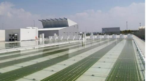
They developed an unique microalgae production system based on photobioreactors. This patented system consists of a number of outdoor closed photobioreactor. These closed photobioreactors prevent any type of contaminants entering the system and in this way they provide high quality microalgae. The systems are monitored and automated, which avoids direct manipulation during harvesting and reduces contamination risks.
